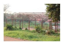
THIS IS A TYPICAL UGANDAN STRUCTURE. BECAUSE UGANDA HAS SO MANY TERMITES, MOST STRUCTURES ARE EITHER STEEL OR CONCRETE.
